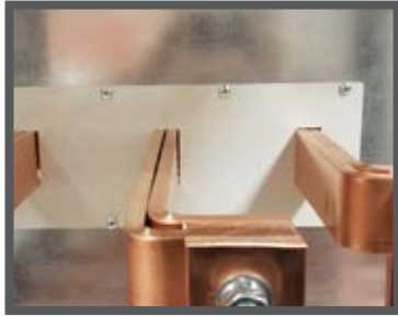
PANO İÇİ GEÇİŞ MONTAGE OF IN PANEL
